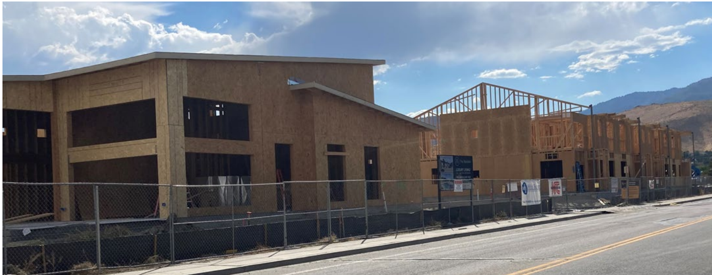
Location: South side Little Lane
